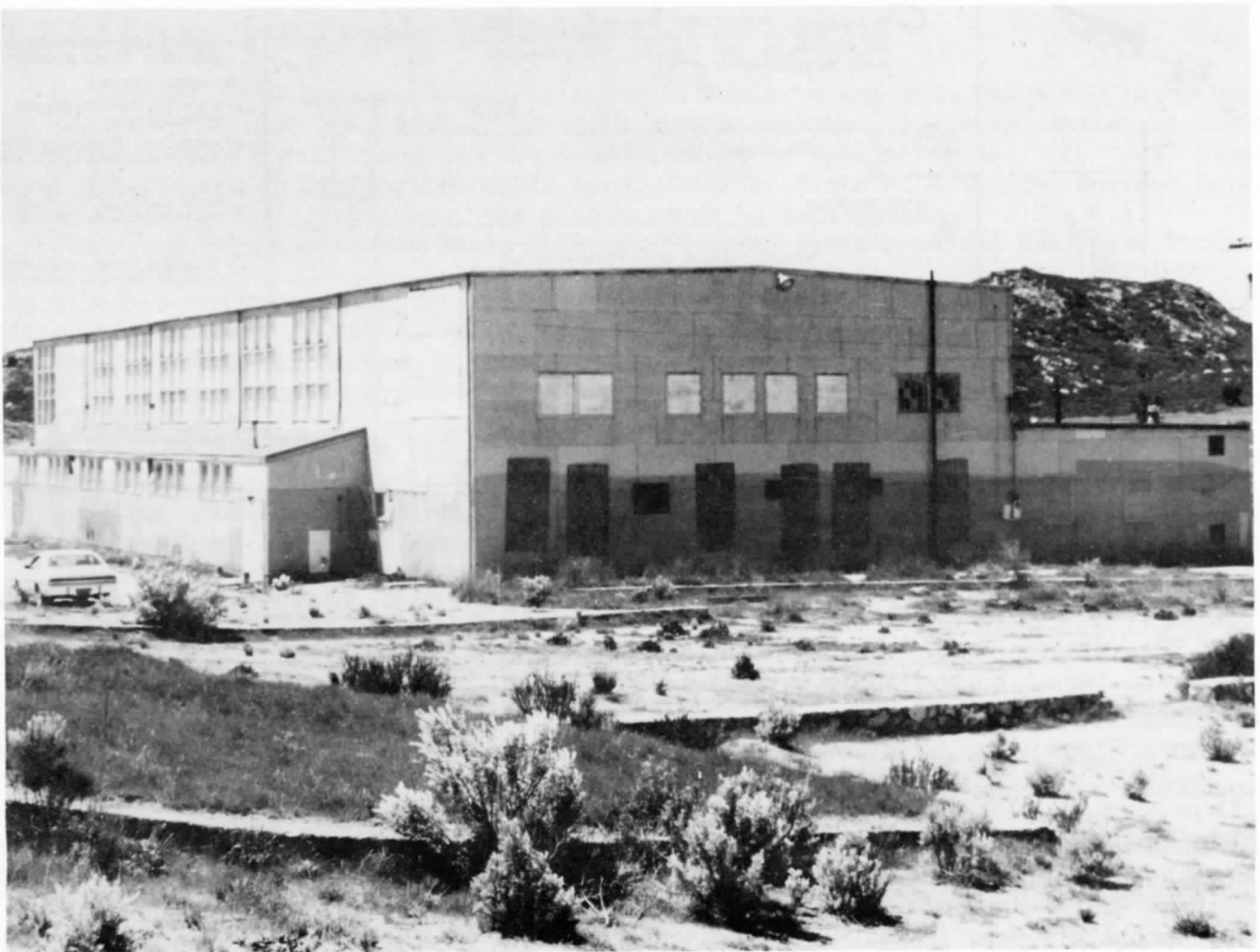
The Campo Creek meadow is shown behind the gym and across the S.D. & A.E. tracks in this view looking west snapped by the REPORT editor last month. The engine house doors will be installed in this end of the building.
